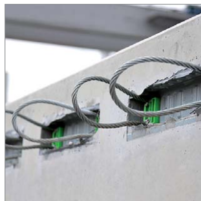
Conectori instalați PFEIFER FS-Box
